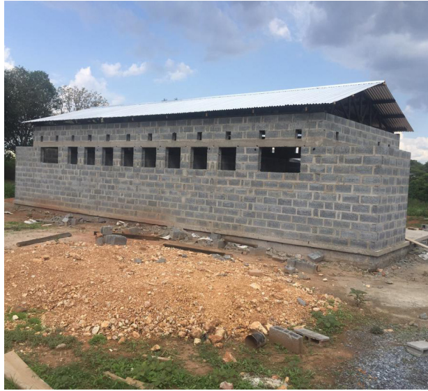
Ablution Block started by 2021 US team in Ndola, Zambia. Roof is now on.
